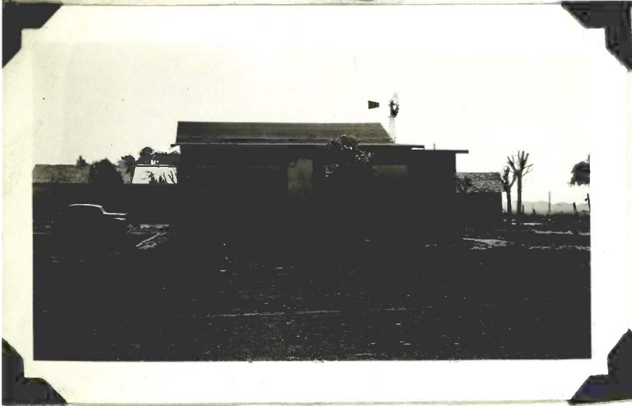
Yard cleared and levelled; trees set out
