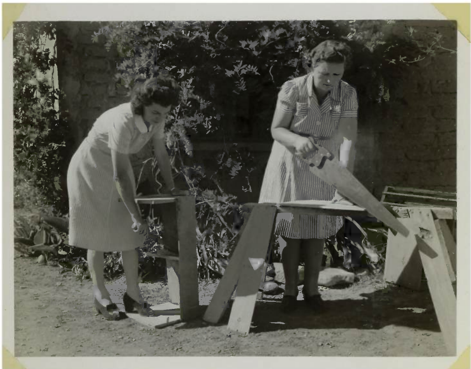
Members of Franklin Homemakers' Club constructing shoe racks from apple boxes.
