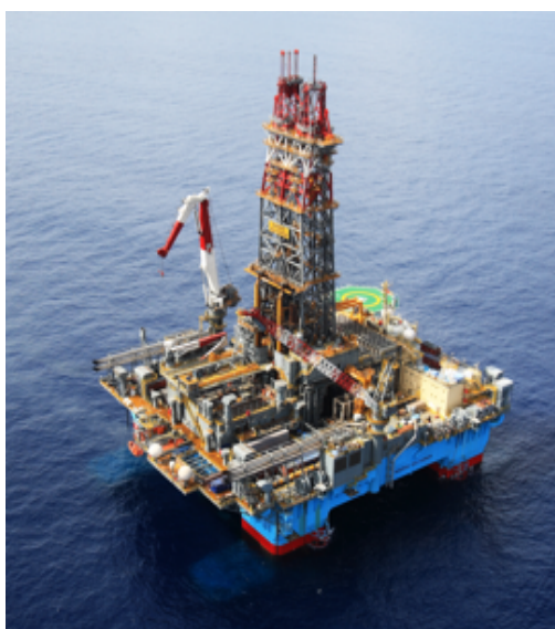
Figure 45: Semi-submersible offshore rig. Source: Maersk.
