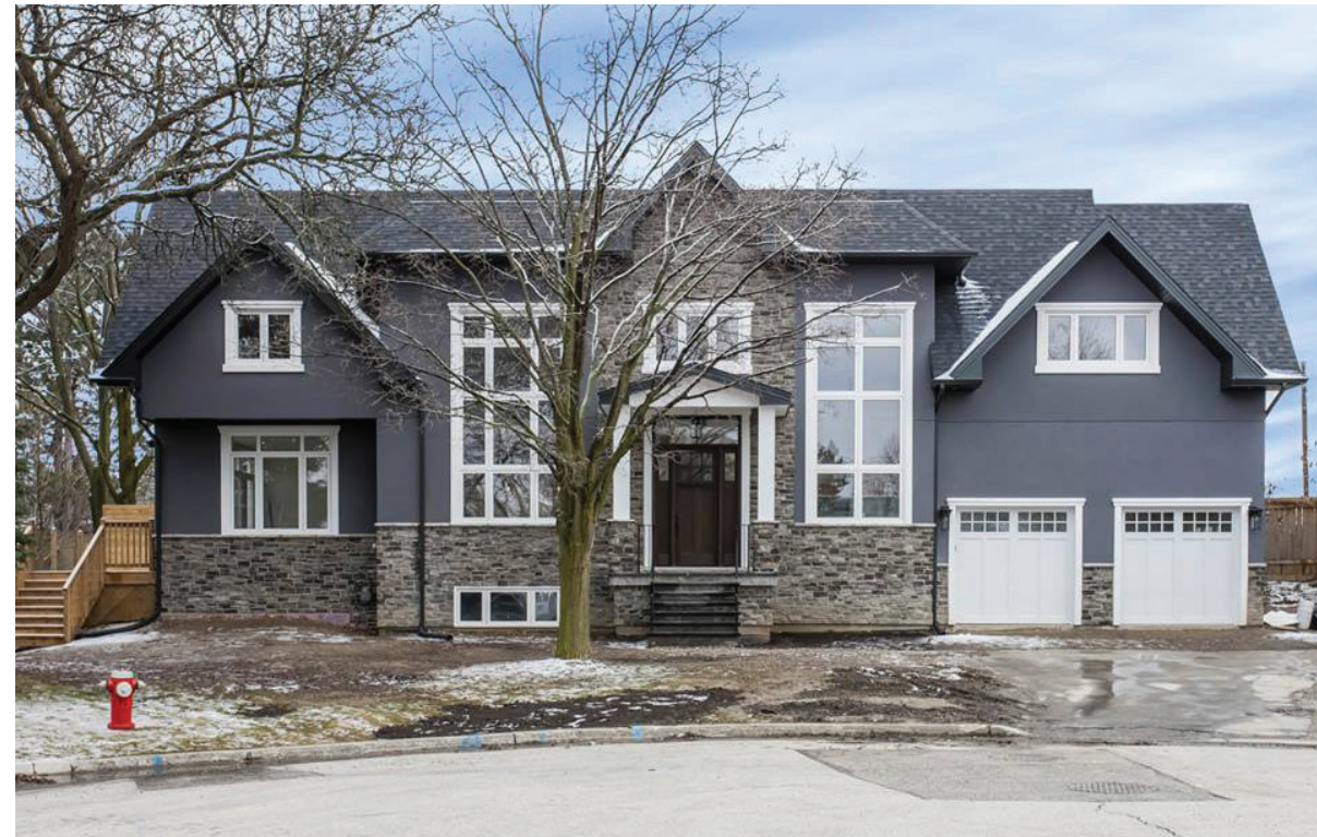
ABOVE: Front Facade of Completed Project
