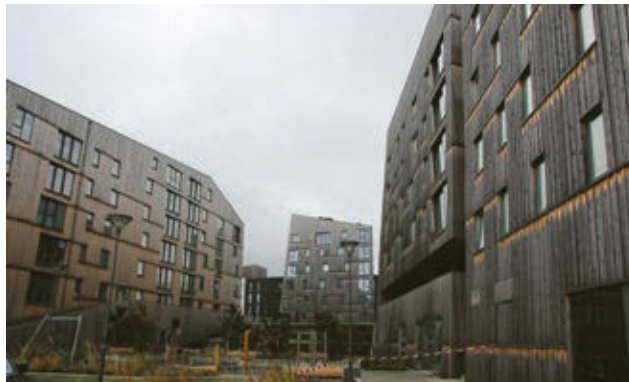
Figure 32: Vannkanten, Stavanger, Norge. Built 2014. Thermally treated pine (Delivered by Moelven). Photo: NIBIO, Ona Flindall
