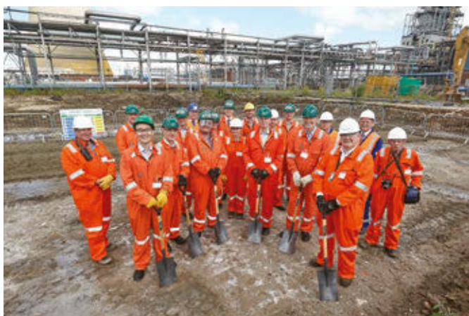
Figure 15: Breaking of soil for new acetylation plant for wood chips at Hull, UK
