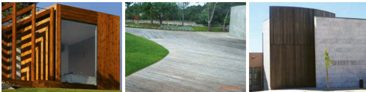
Figure 35: Examples of imported modified wood in use in Portugal. From left: Treehouse in Duoro (ThermoWood), Decking at Buçaquinho (Plato), and Cladding in Penafiel (Kebony)
