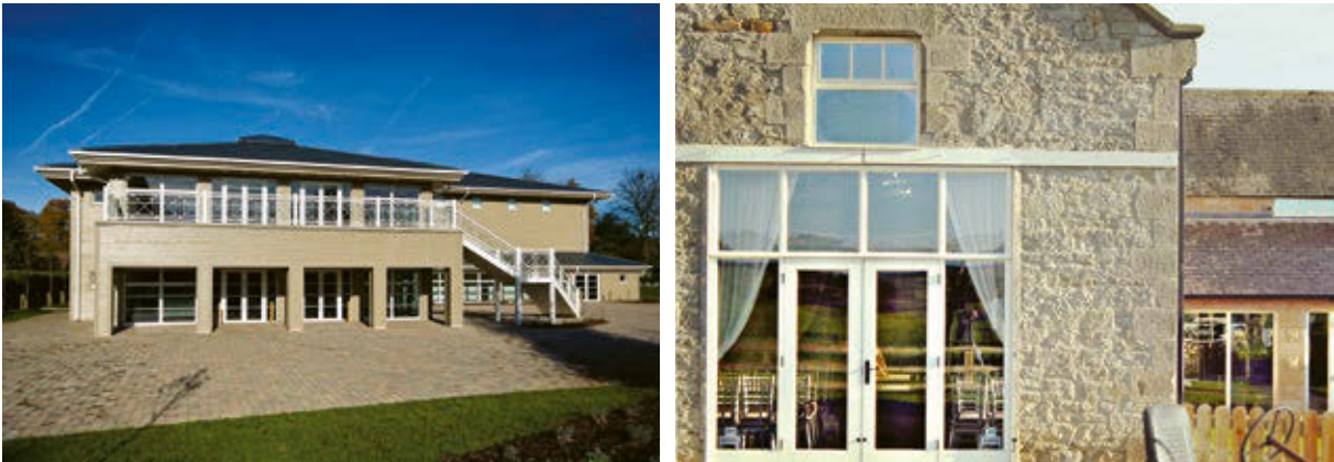
Figure 46: Accoya cladding at Pipers High School London (left), and the joinery company Richard James in Northumberland, UK
