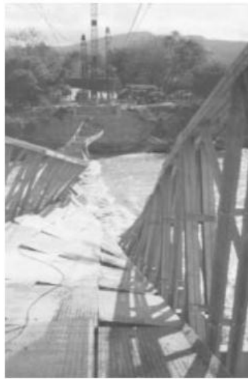
(c) Puente Los Angeles
