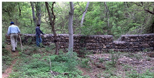
Fig. 4. A working gabion check dam in the Culiacán watershed (Mexico).
