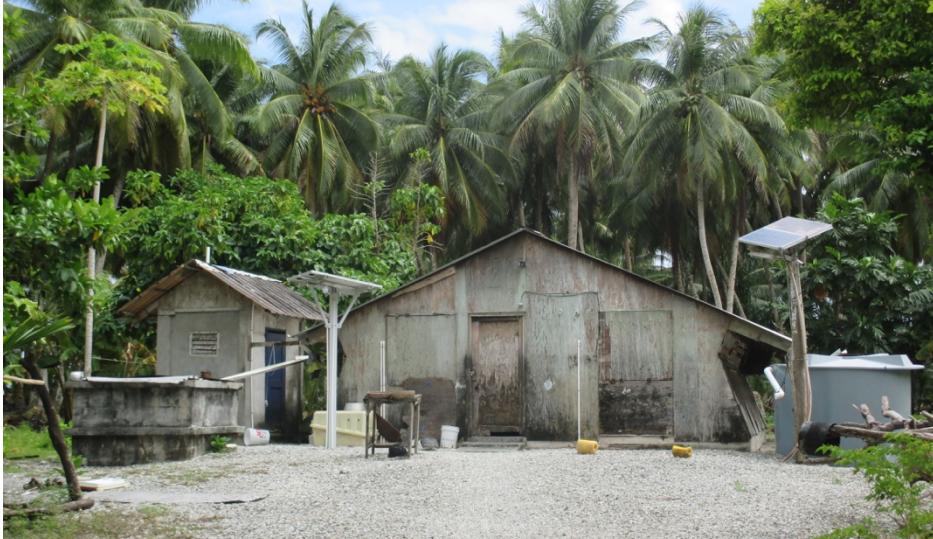
Figure 5. Post-disaster shelter deployed by FEMA after Typhoon Alice devastated Namdrik and Jaluit atolls, RMI. This wood framed structure with concrete slab on grade, is a one room dwelling used primarily for sleeping and crafts making.
