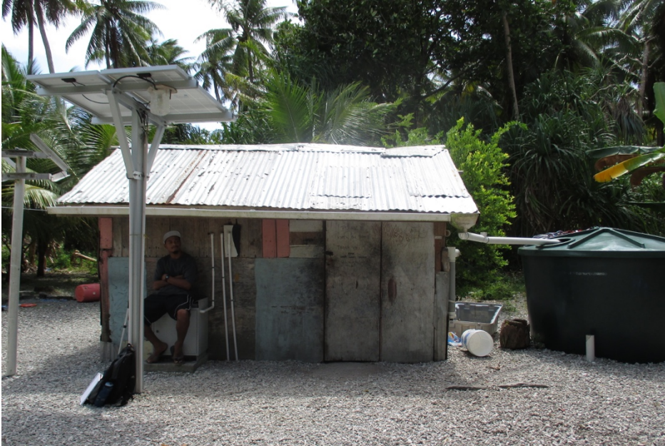
Figure 7. A typical self-built dwelling on Namdrik, which is similar to self-built dwellings found on Majuro. It is constructed of recycled imported building materials and used primarily for sleeping.
