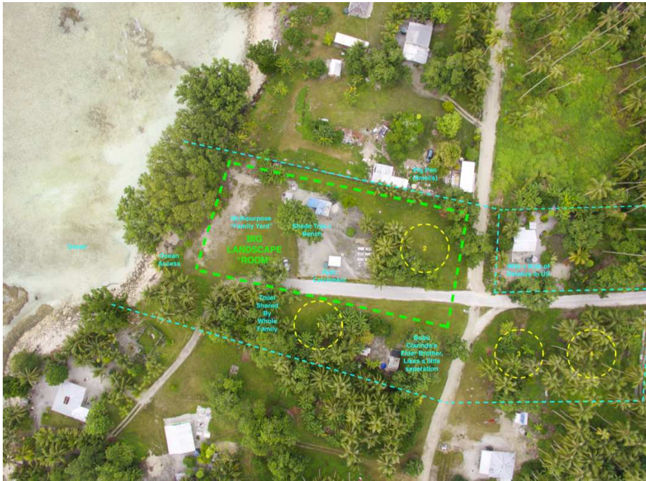
Figure 11. Aerial image of the specific site with approximate boundaries. The coral spread is evident in the center of the green rectangle. This was the location of the house that burned down.
