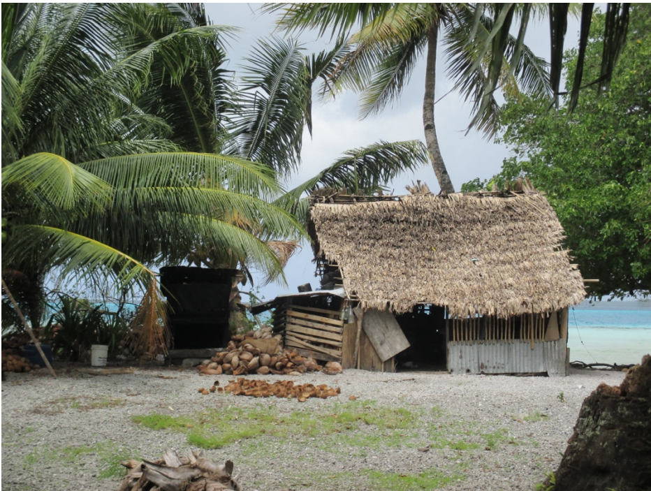
Figure 8. A typical cook house constructed primarily of local materials as evident in the pandanus paneled roof.
