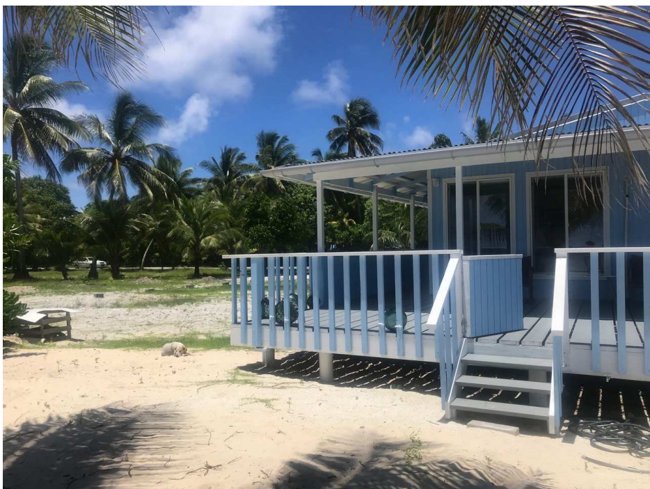
Figure 9. Photograph of house completed in 2019 in Majuro, RMI constructed of PVC pier foundation and wood framed construction. It demonstrates slight innovations in housing design for Majuro.
