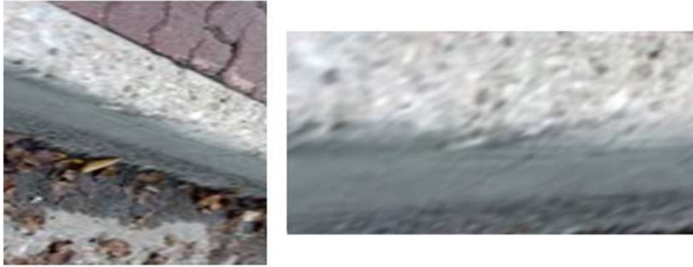
Fig. 4.16. Pattern 1. Real curb (Left), Example Pattern of 6 inches Wide, 6 inches Tall and 24 inches Long (Right).
