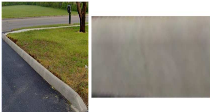
Fig. 4.23. Pattern 5. Real curb (Left), Example Pattern of 6 inches Wide, 6 inches Tall and 24 inches Long (Right)
