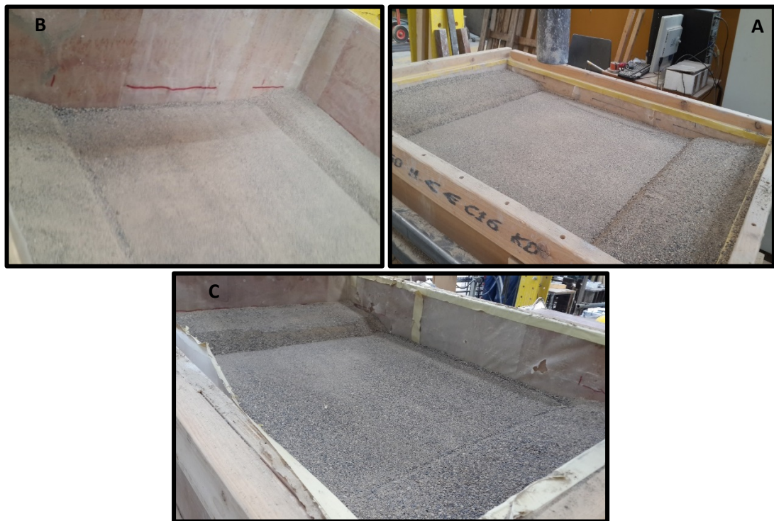
Figure 6.29. Soil surface settlement after removing the applied loads of unreinforced embankment (A) 200 mm (B) 400 mm and (C) 600 mm.
