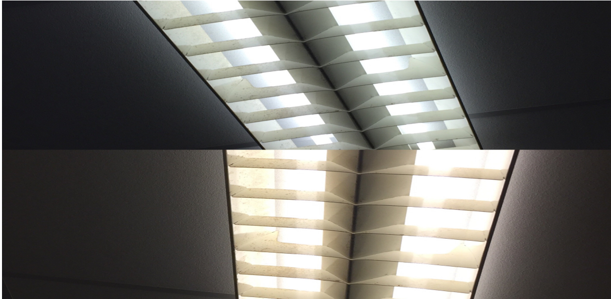
Figure 3.3. Classroom light bulbs before and after modification (6500K baseline A1 and A2 to 3000K intervention B1 and B2).
