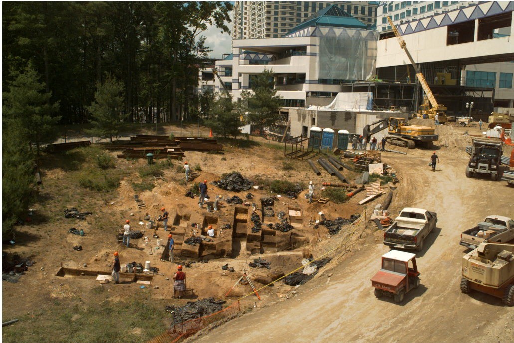
Figure 1.4, Summer 2006 excavations in preparation for West Access Road.
