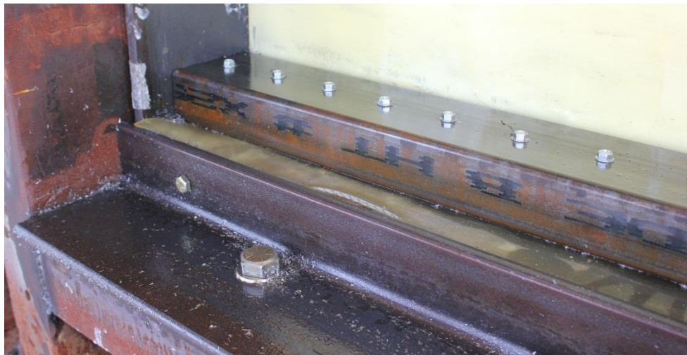
Figure 27: Bottom Tube Clamping Polyurea Sheet
