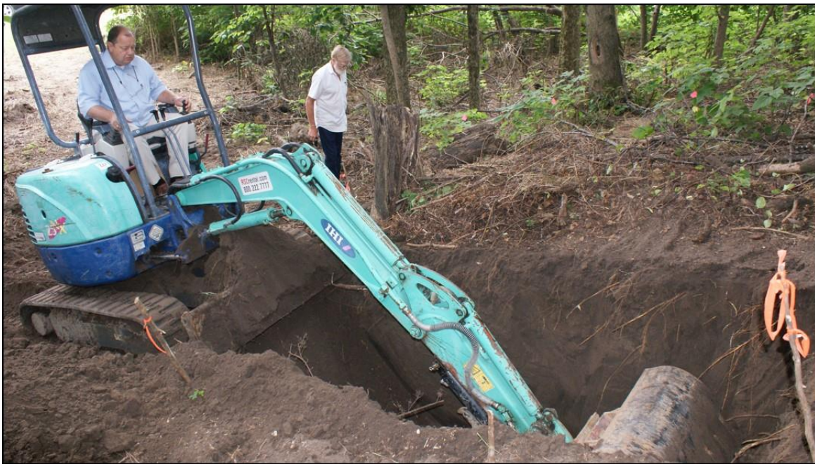
Figure 16. Trench being excavated
