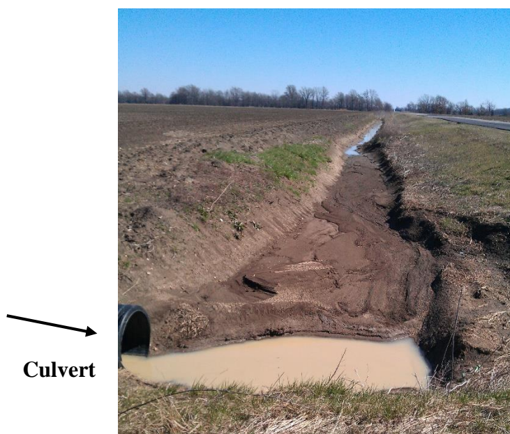
Figure 14: Culverts collecting water near the fields in the Howden Lake watershed
