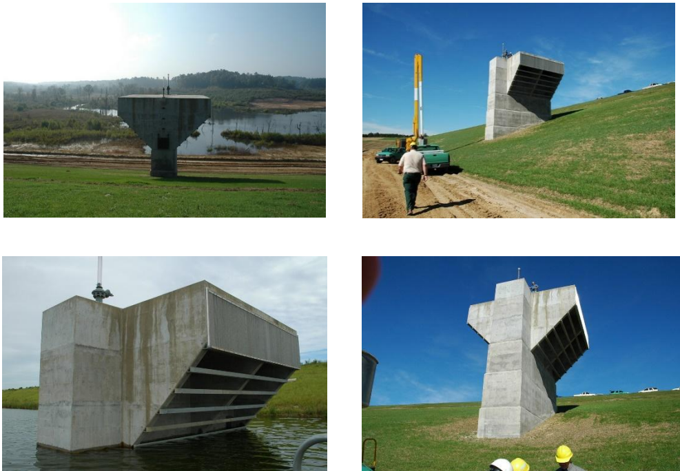
Figure 2.6: Final concrete box conduit (Bingham, 2014).
