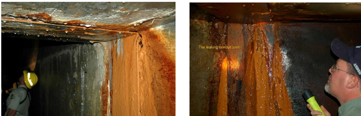
Figure 2.5: Box conduit inspection (Bingham, 2014).
