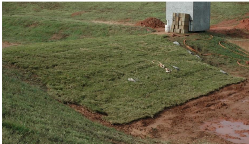
Figure 3.2: Picture of the model embankment dam.
