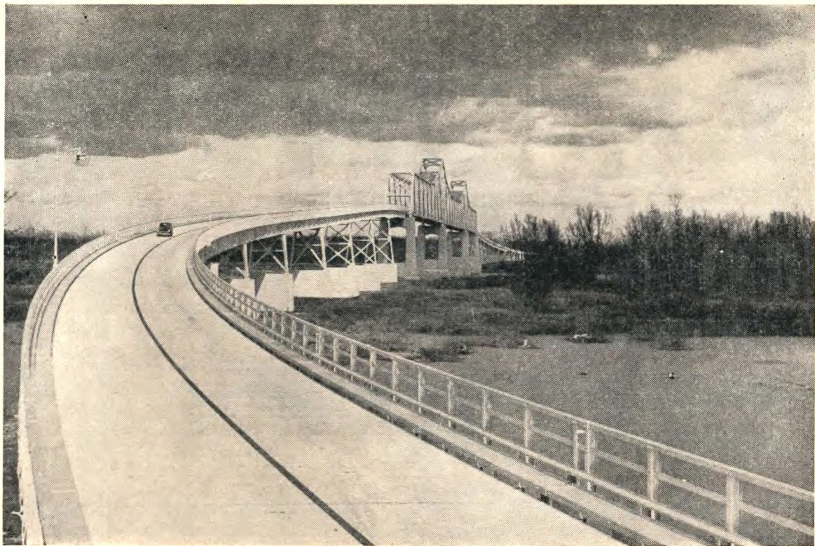
GREENVILLE-LAKE VILLAGE BRIDGE OVER MISSISSIPPI RIVER
