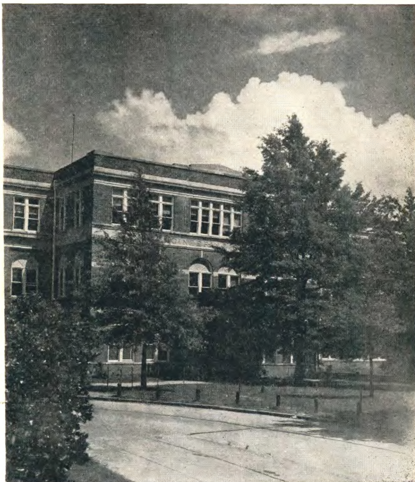
Engineering Building, Mississippi State College
