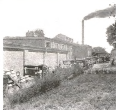
CONDENSED MILK PLANT STARKVILLE
