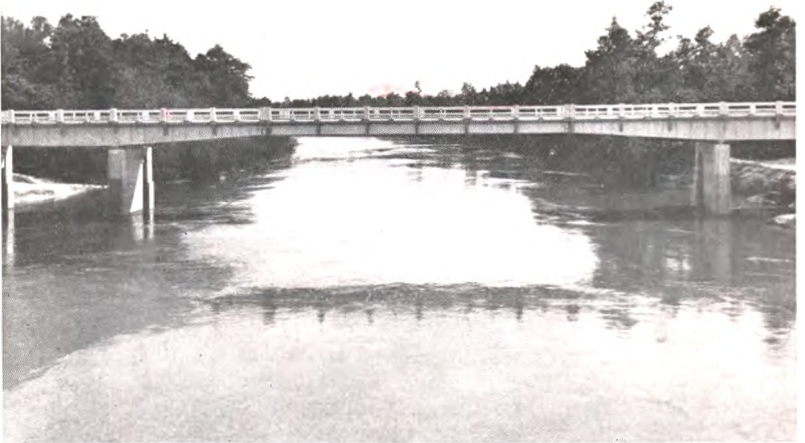
STEEL AND CONCRETE BRIDGE
