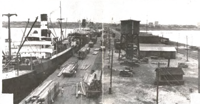
DEEP WATER PORT - GULFPORT
