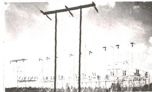
ELECTRIC POWER - GREENWOOD
