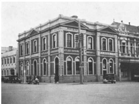
FIG. 2: Reed Building, corner of Jetty and Crawford Streets, Dunedin. Alfred H. Reed, A. H. Reed: An Autobiography , A.H. & A.W. Reed, Wellington-Auckland-Sydney, 1967, p.127. Reproduced by permission of Alfred and Isabel and Marian Reed Trust.
