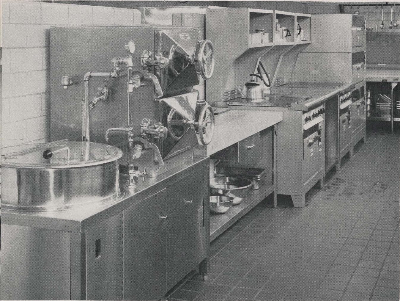
Electric steam cooking has proven to be a fast, economical operation for school cafeterias.
