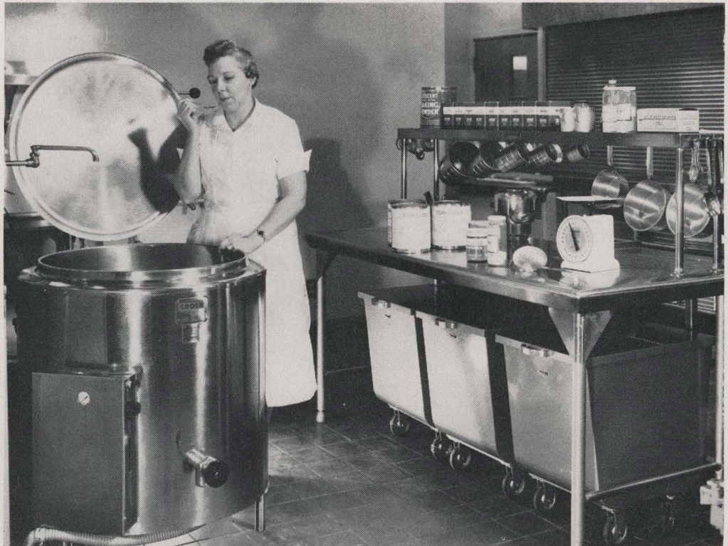
Steam-jacketed kettles are heated electrically and require little maintenance.
