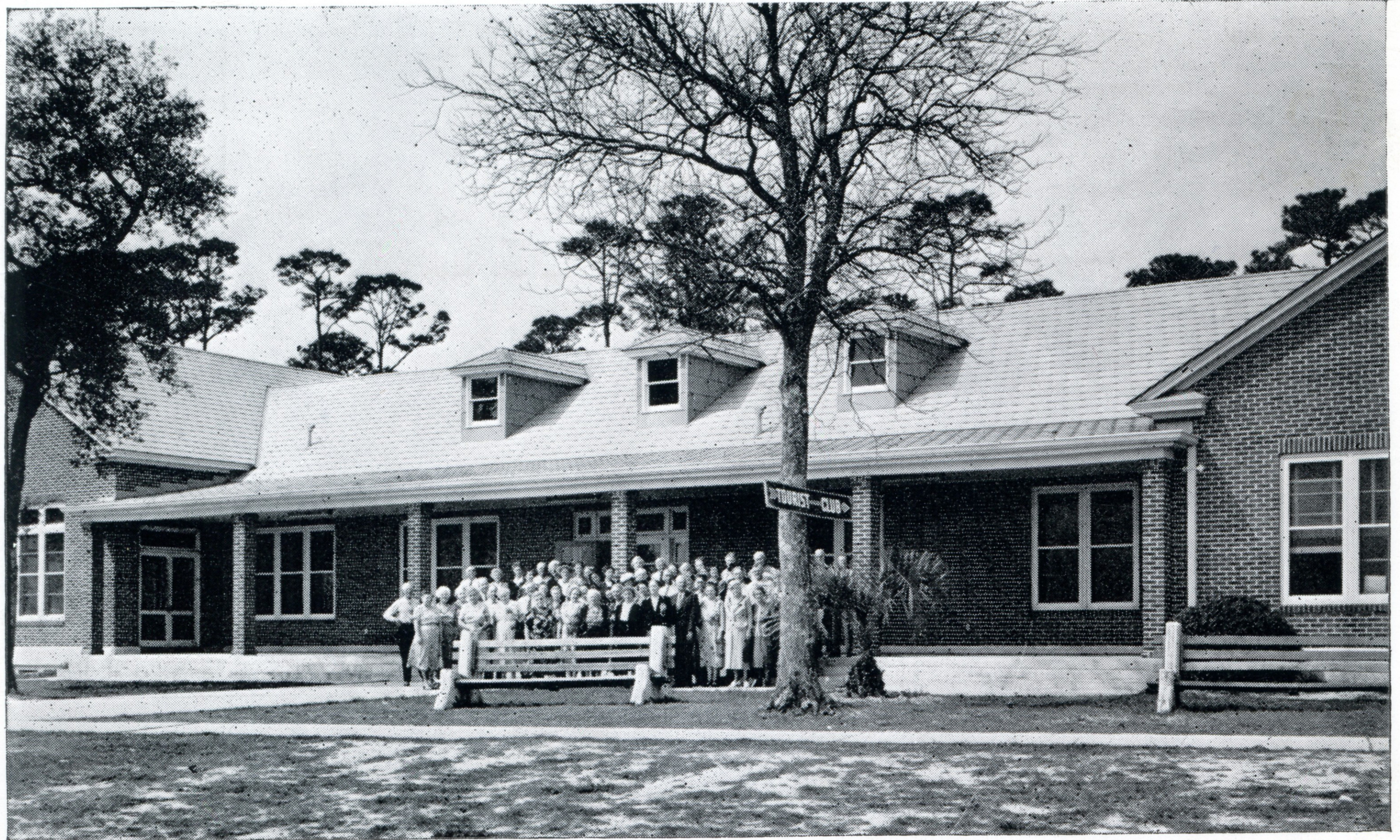
WEST SIDE COMMUNITY HOUSE . . . WEST BEACH . . . GULFPORT, MISS.
