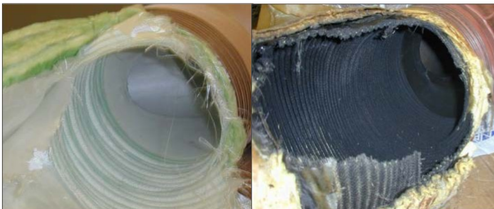
Figure 3.2 Duct sections inspected by UK Civil Aviation Authority (CAA 2004)
