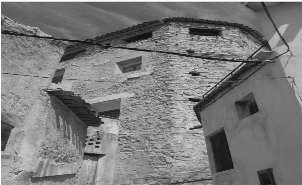
Figure 14: Stone masonry in detail
