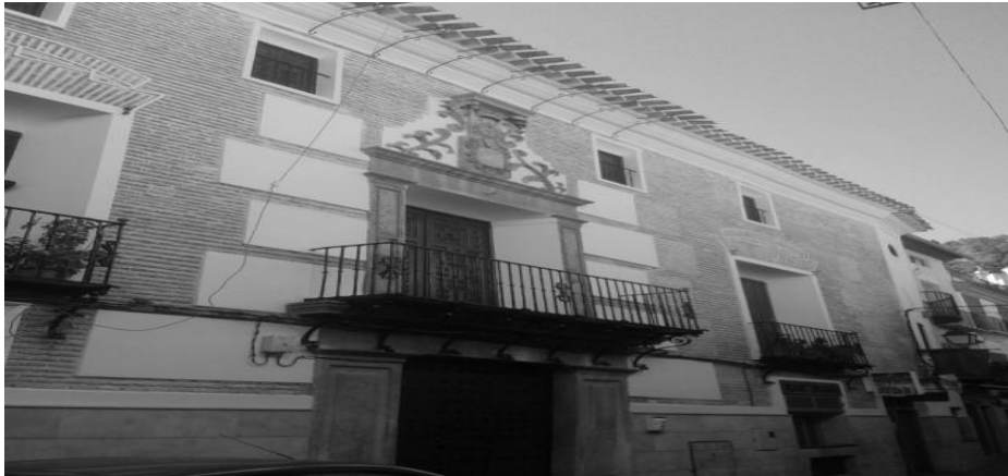
Figure 13: Image of a building in Main Street, 52
