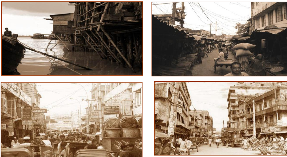
Photograph 1: Existing set up of Boro Bazaar area (Ahsan & Rahman, 2005)
