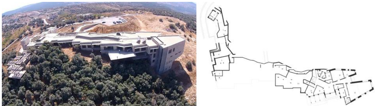
Fig. 5 Emphasized the aesthetic and environmental value of integrating architecture with nature through the organic outer walls. Source http://ohkconsultants.com
