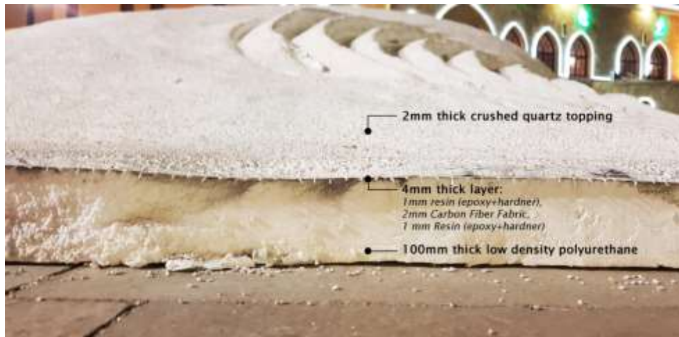
Fig.8: Structural and Finishing Layers of the structure Reference: Photographed by the authors - July 2018
