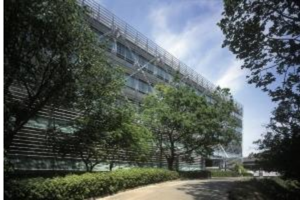
Figure 2.3 - RC building retrofitted with steel braces (Tokyo Institute of Technology)
