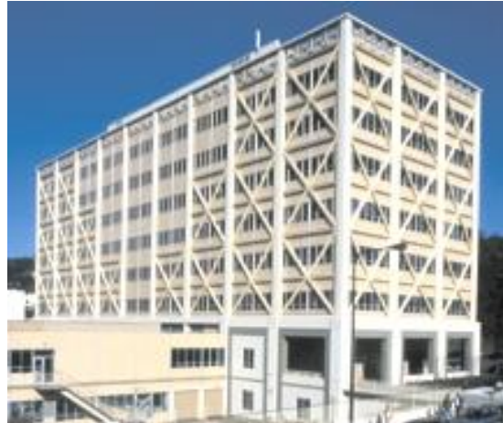
Figure 1.3 - Seismic retrofitting of RC buildings with steel braces
