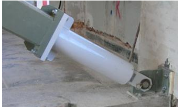
Figure 2.7 - Example of a dissipative device applied in BRB
