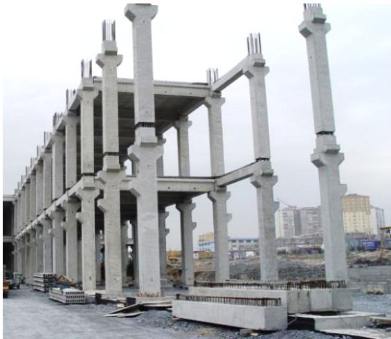
a) Dowel beam-to-column connection [20]
