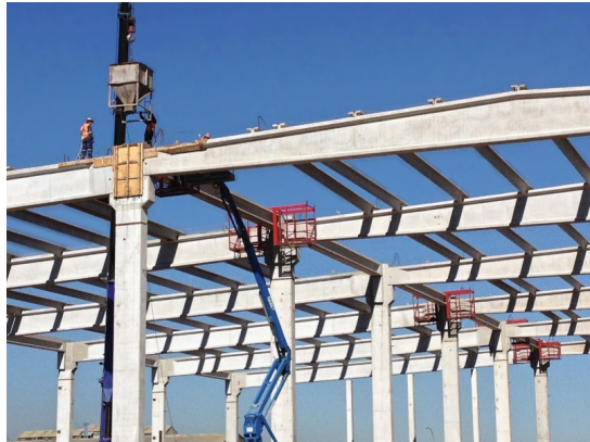
a) Casting of the beam-to-column connection [15]
