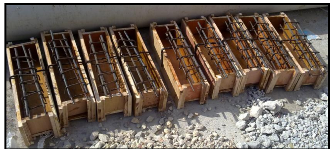
Figure (2): The moulds before casting of concrete
