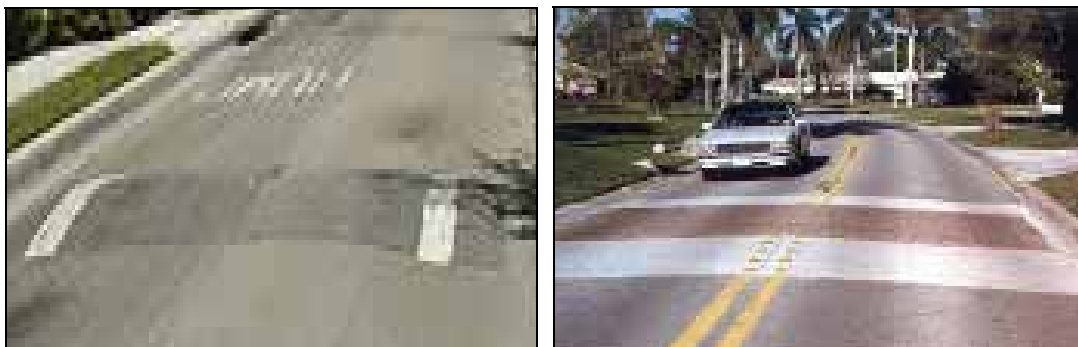
Figure (51) Traffic Calming - Vertical speed control measures
