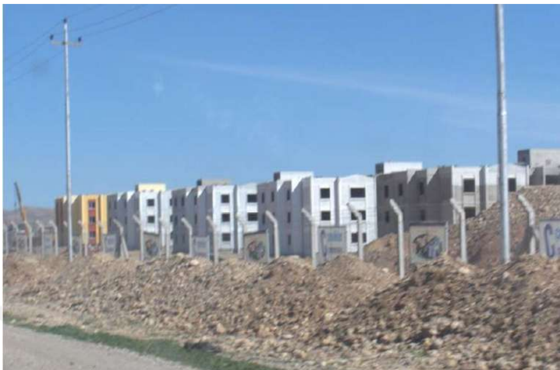
Figure A.3: Residential Units Under Construction
