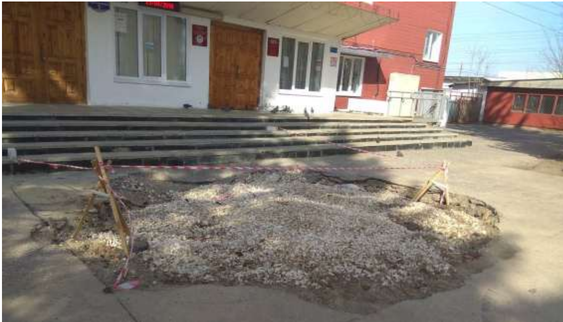
Figure 10: The hole in the flow of suffusion processes
