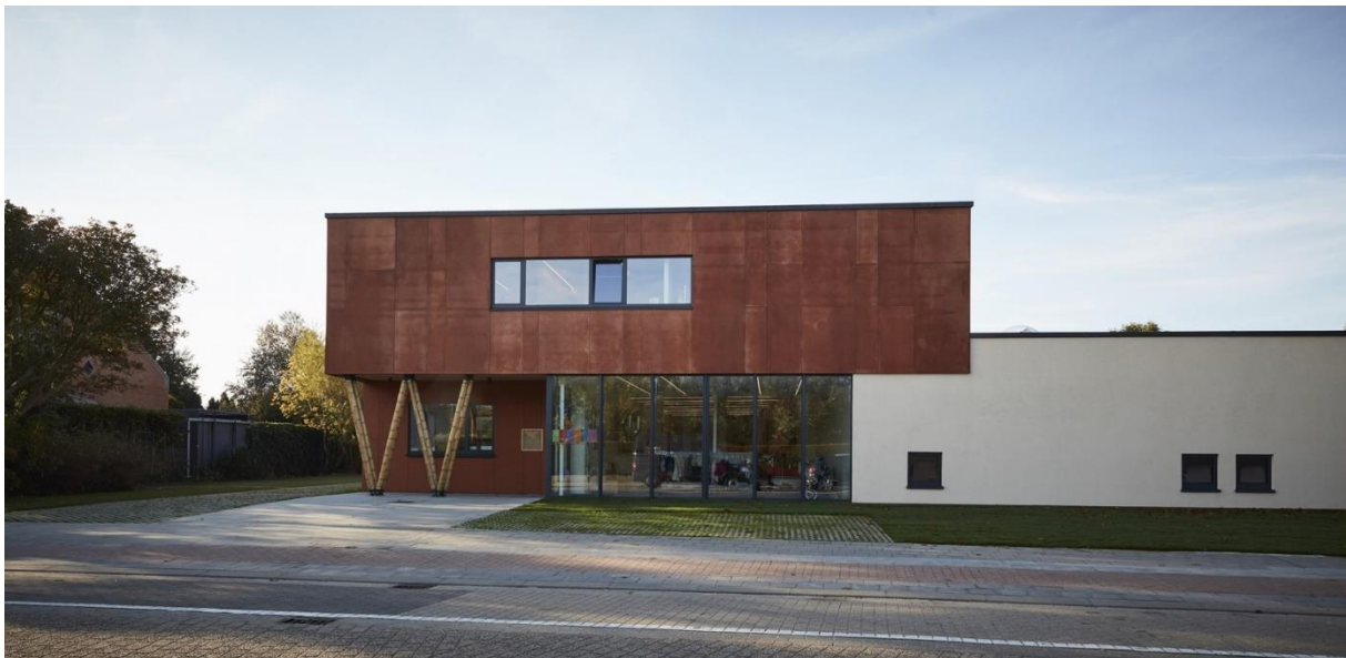
Pic. 21: Front view of Daycare center Wiegeliel [55]
