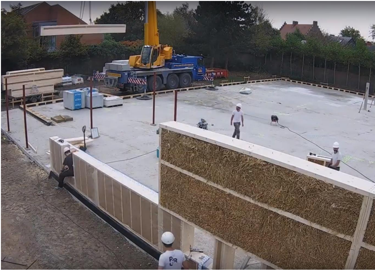
Pic. 23: Assembly of panel boxes filled with hemp [55]
