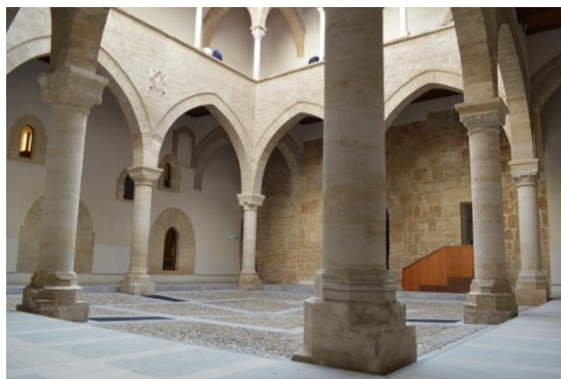
Figure 9. The inner courtyard.
