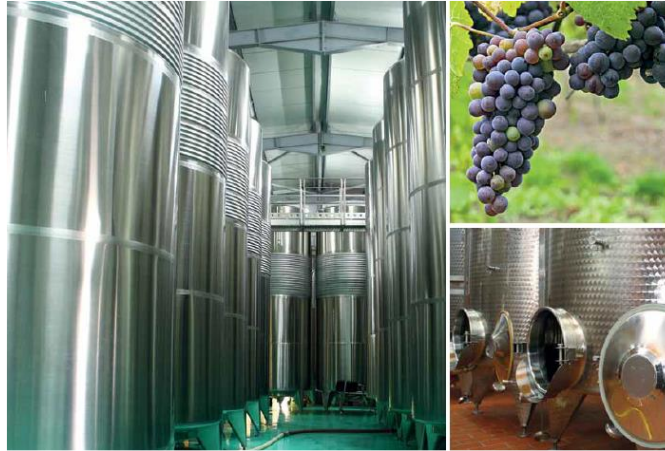
Fig. 2-5. Wine storage tanks 45 .
