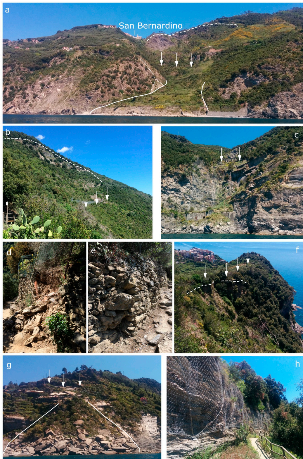
Figure 4. Main landslides and critical issues recognized along the “Sentiero Verde-Azzurro” trail: (a) Guvano landslide; (b) Macereto area; (c) rock sea cliff equipped with falling rock protections, Crovarla Valley; (d) local dry-stone wall collapse along the path; (e) visible dry-stone wall deformation along the SVA trail between Vernazza and Corniglia; (f) degradation scarp in correspondence of the Guvano beach, close to Corniglia; (g) rockslide close to Vernazza; and (h) local rock falls corresponding to the bedrock outcropping along the “Sentiero Verde-Azzurro” trail. White arrows indicate the path location.
