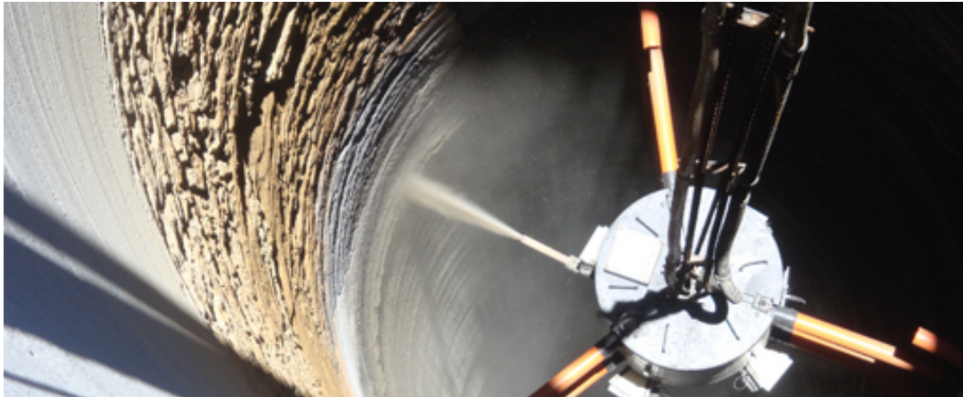
Figure 8: Robotic shotcrete machine in a ventilation shaft
