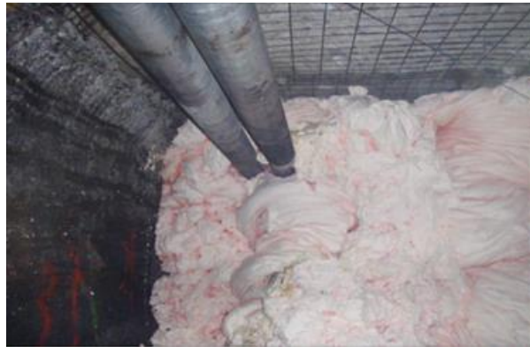
Figure 11: Example of a ROCSIL® FOAM seal forming around mine infrastructure
