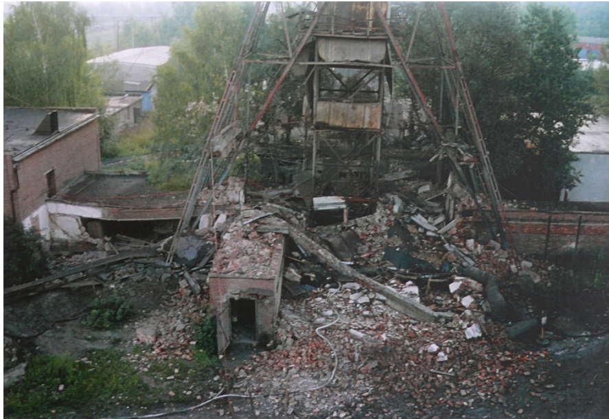
Figure 1: Gas explosion at Hermanice Mine during the liquidation of the He-III shaft
