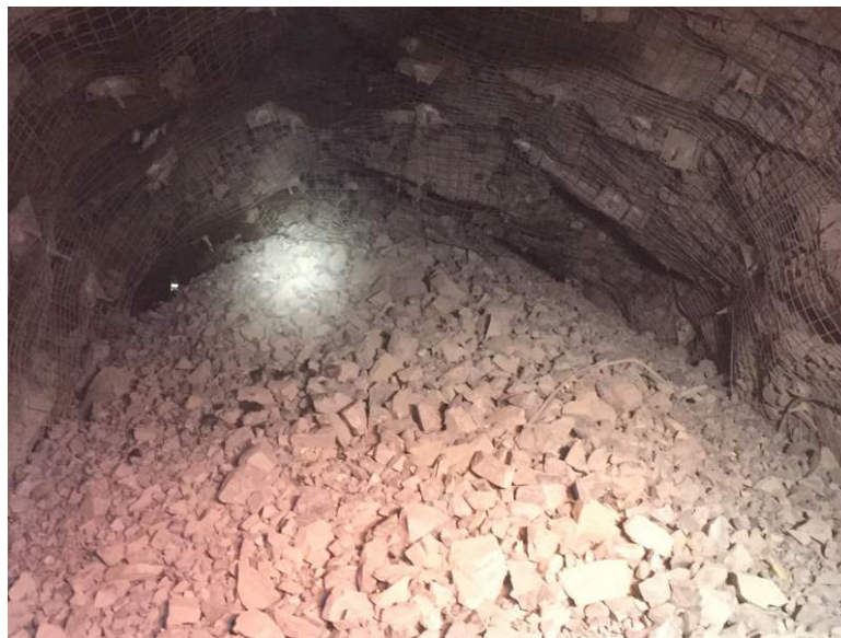
Figure 11: 9700 OD01 R59 bogging with precharged R61 not visible
