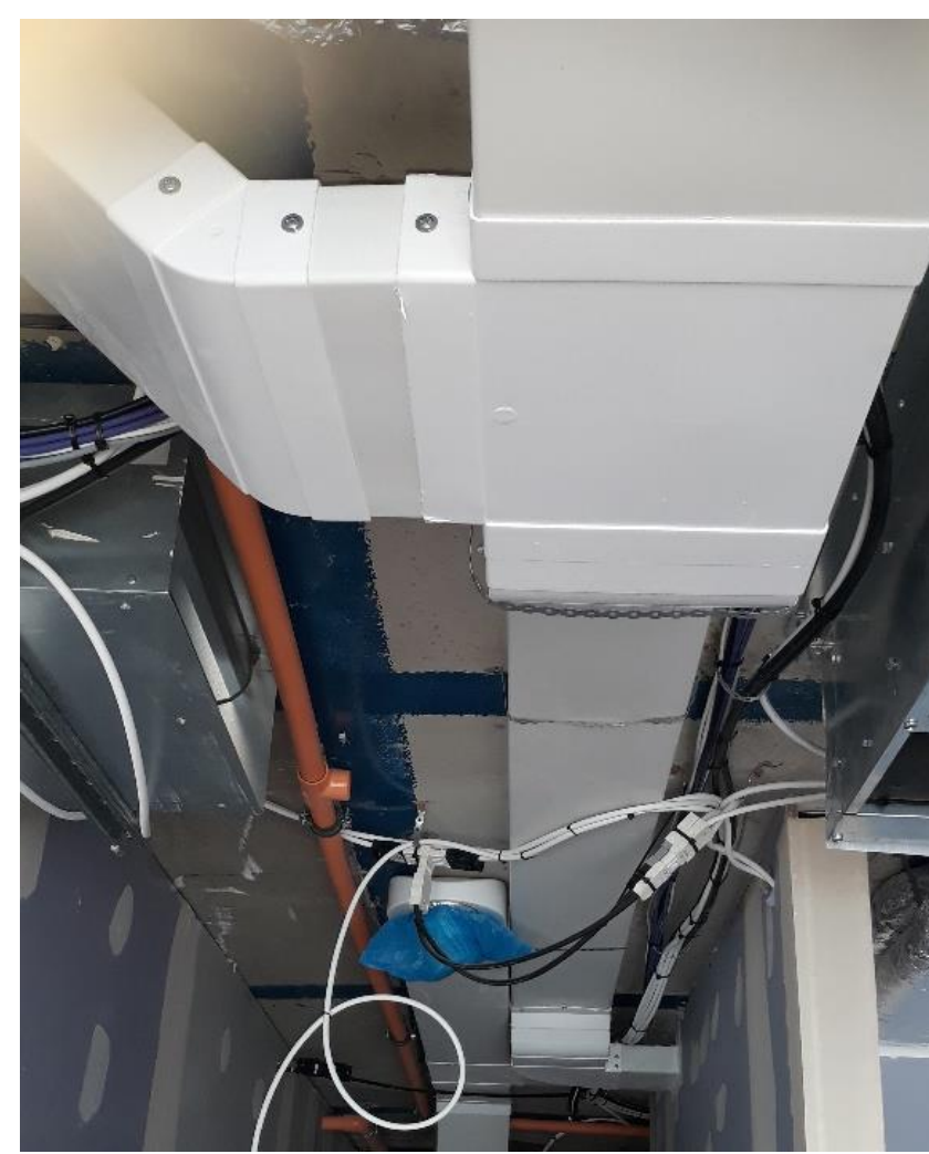
Fig 2. Typical plastic duct T-Branch
