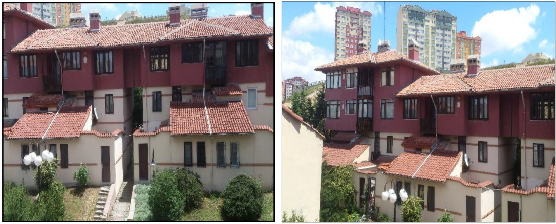
Figure 7.33: The top roof form of the Eryaman Third Stage project. Source: the researcher.
