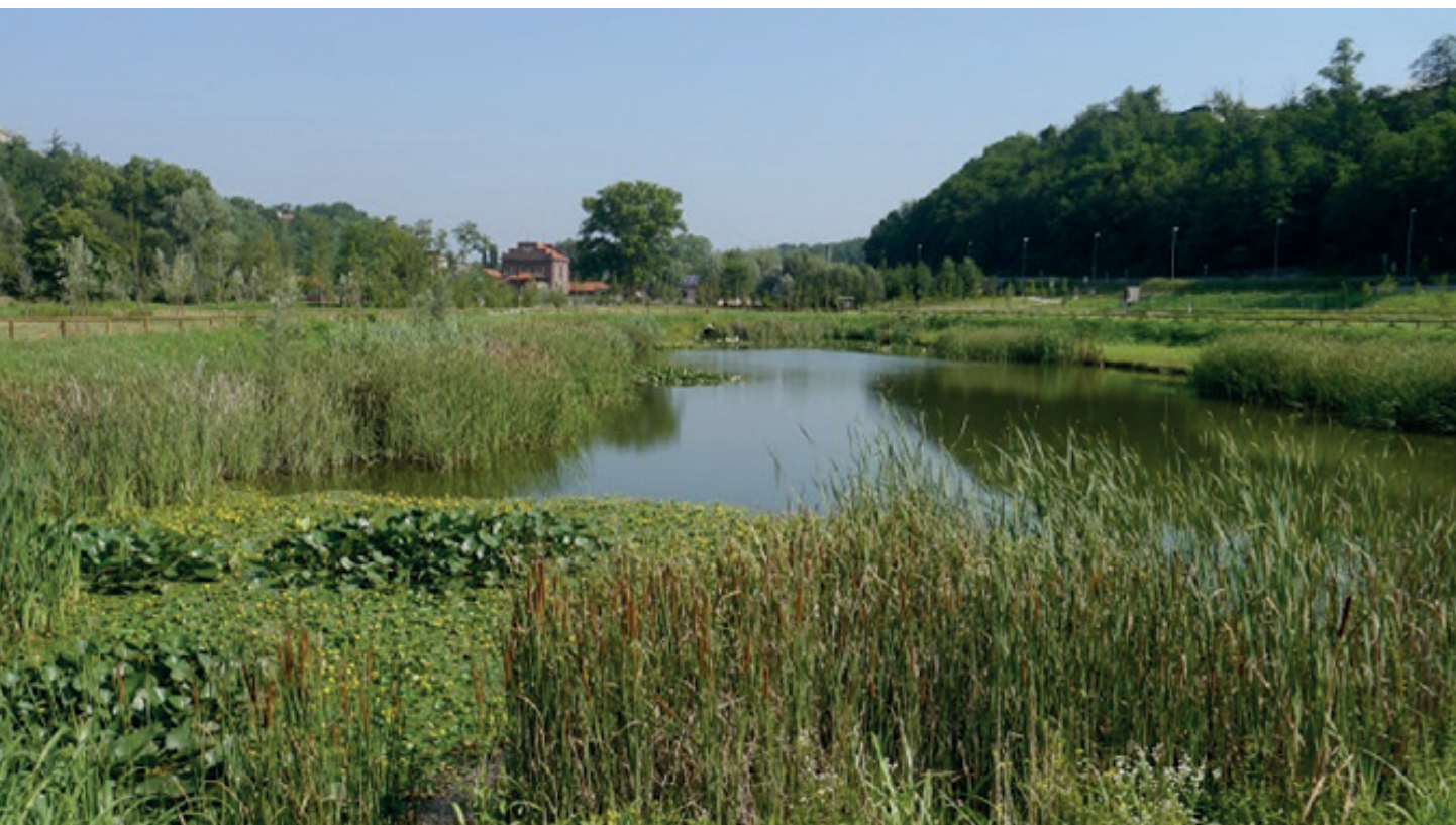
Figure 5.17. Constructed wetland in Gorla Maggiore, Italy ( https://oppla.eu/casestudy/17252 )
