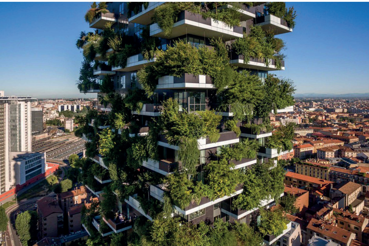
Figure ES.1. Vertical Forest realized in the centre of Milan, credited to the architect Stefano Boeri ( https://oppla.eu/casestudy/17625 )
