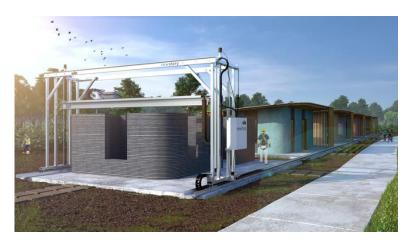
**Figure 1.** A 3DP construction of houses on a railing system **Source:** iconbuild.com
