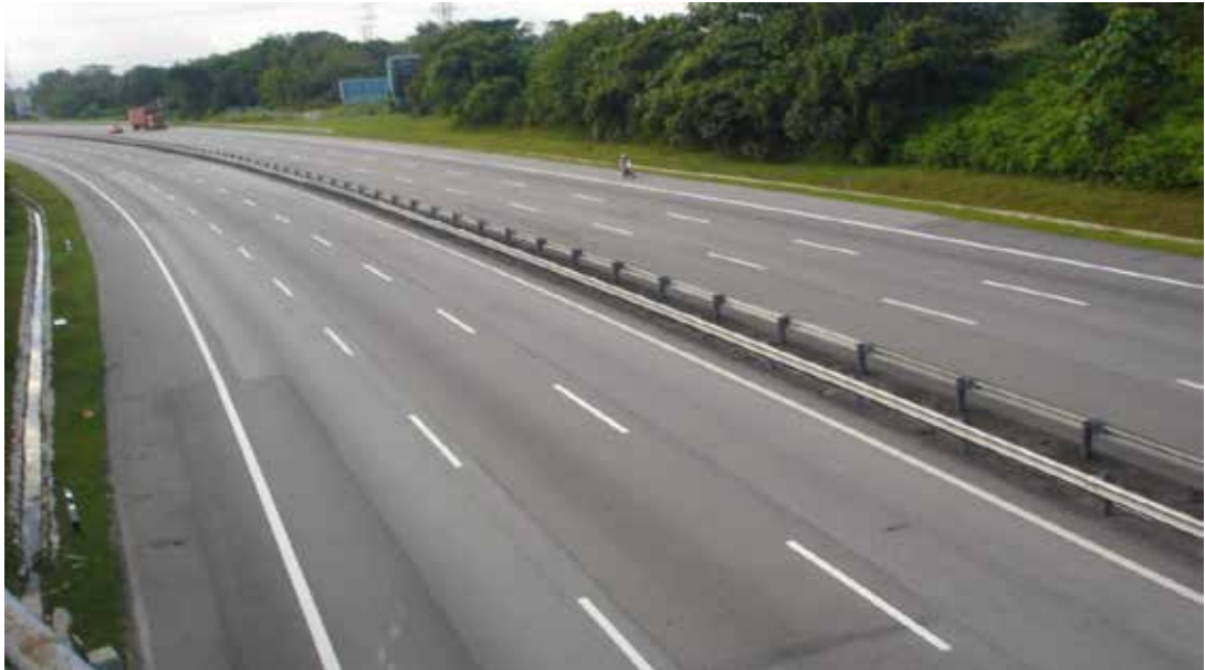
Plate 1.2: Typical 6-lane basic segment expressways in Malaysia
