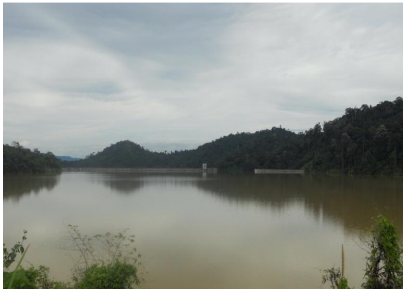
Figure 1.2(b) SASD reservoir
