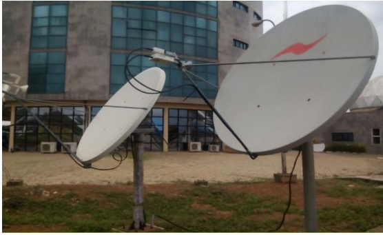
Figure 3. Broadband VSAT Outdoor Unit Receiving on the Ku-Band Frequency from Nigcomsat-1R.
