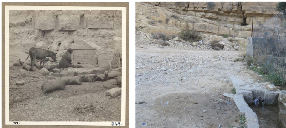
Figure 3. 'Ayn eṣ-Şader in 1930 (left) 4 and in 2018 (right)
