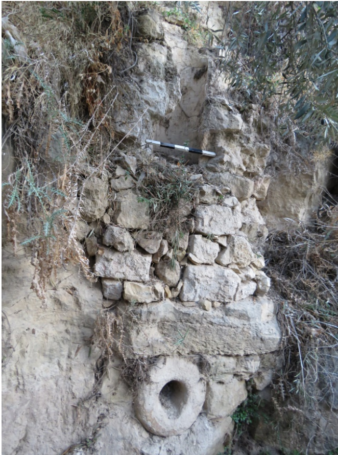
Figure 10. Image showing the remaining part of Mill 3
