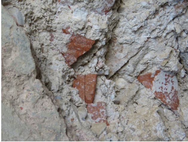
Figure 12. Image showing the pottery sherds that were mixed with the mortar applied to Mill 2
