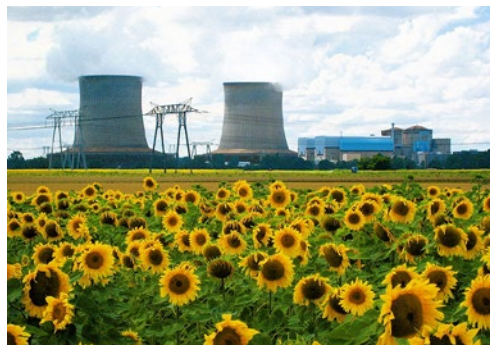
Image 68, Centrale-nucleaire-Saint-Laurent-des-Eaux (2007). photo by Nitot (CC BY-SA 3.0)
