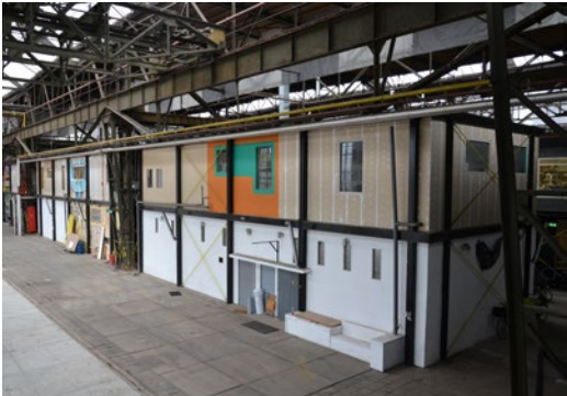
Image 110, former shipbuilding shed turned into workshops, Amsterdam. Pers. Archive, 2014-10-07
