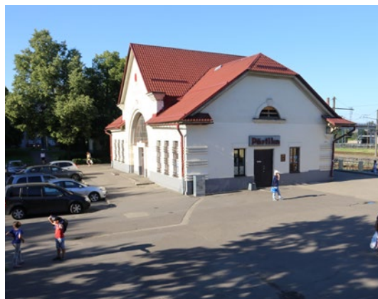
Image 149, Existing train station. Field Study, 2017-08-10
