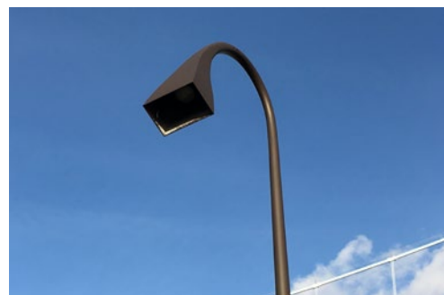
Image 202, Street lighting , Gothenburg, Sweden Personal Archive, 2016-09-22
