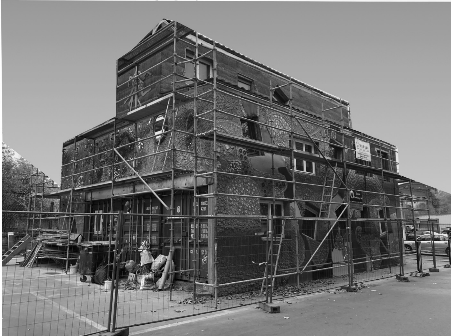
Figure 4: BENU Village under construction
