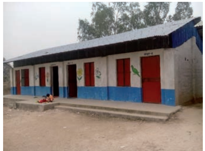
Figure 2. Typical one-story brick school building (source: SAFER, 2019a).
