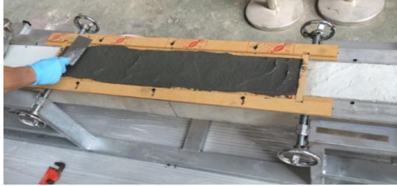
(b) First layer of cementitious matrix
