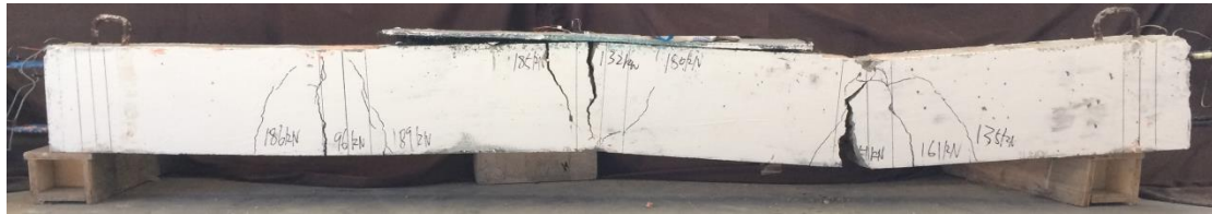
(b) Beams strengthened on the hogging moment region (CB-C-F2-I40-T)
