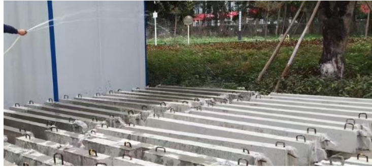
Fig. 3. Accelerated corrosion of specimens using wet-dry cycles
