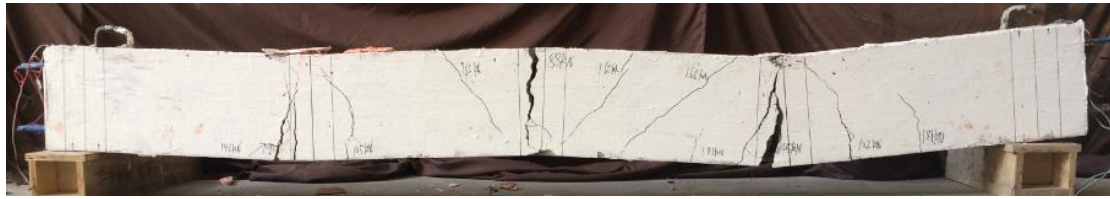
(a) Unstrengthened beams (CB-RF)
